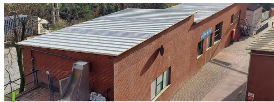
Renovated Treatment Plant - 2021
